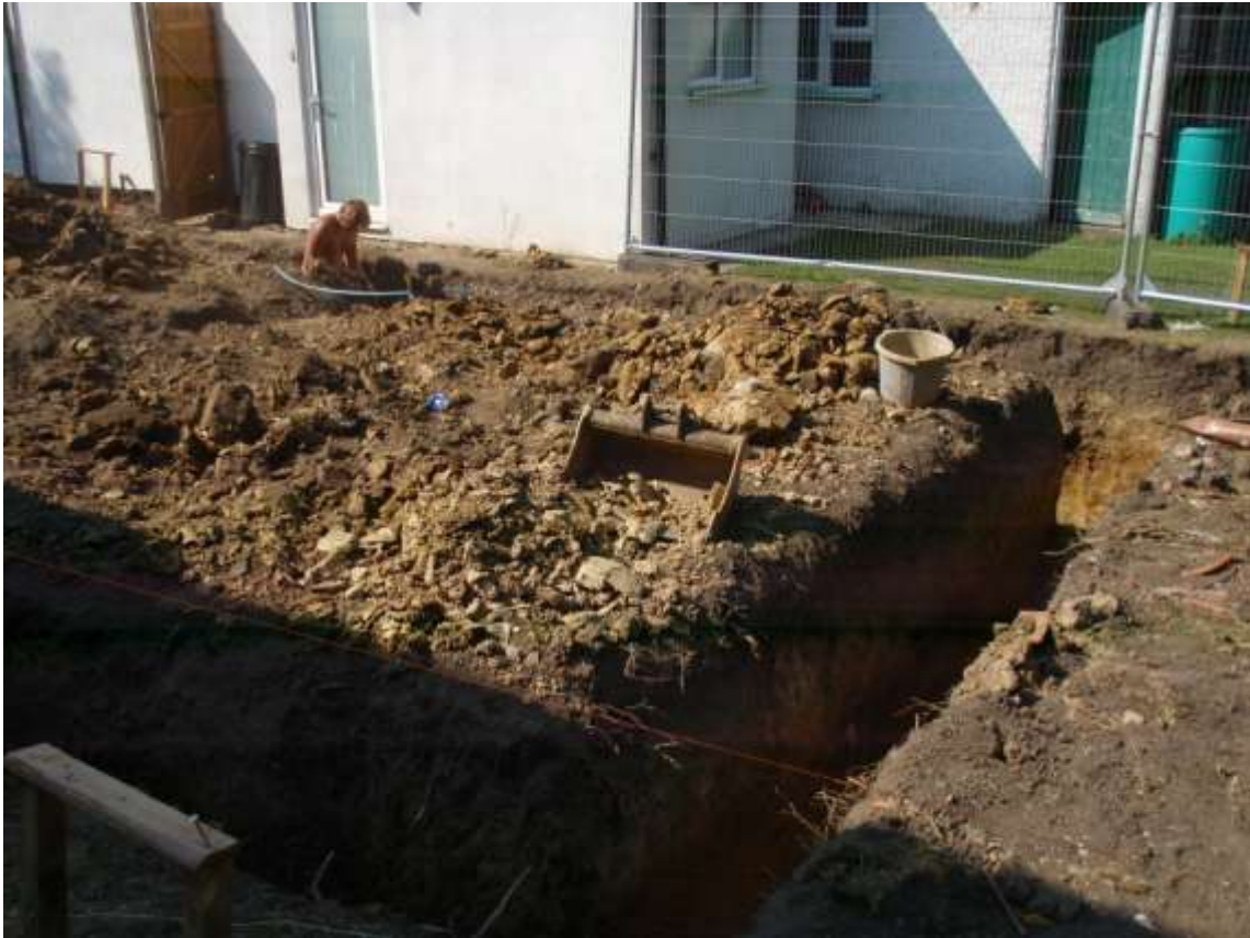
Plate 2. General view of site (looking NW)
