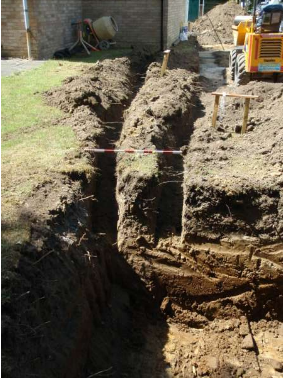
Plate 7. Drainage and service trench (looking E)
