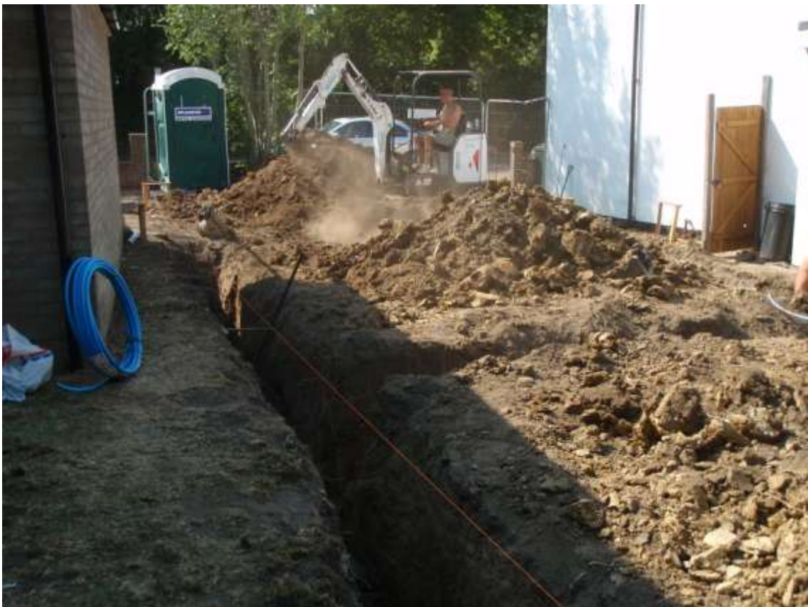
Plate 3. View of foundation trenching at entrance (looking W)
